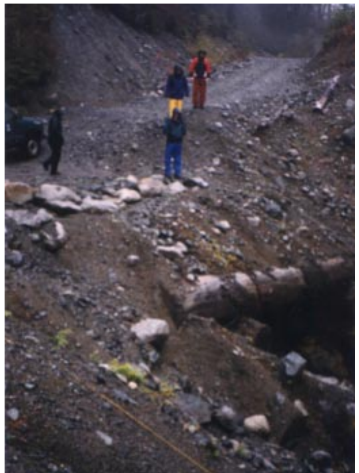
Figure 26. Site 45 after road deactivation. There is evidence of past rill erosion, but the deactivation has diverted water away from the crossing.
