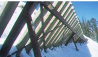
FIGURE 68 Snow support structures built in an opening above a subdivision, Big Sky, Montana. Forest is slowly regrowing between the structures. Such works require professional engineering design in British Columbia.
