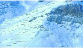
a) A network of rigid snow-supporting structures installed to resist snow avalanche initiation.
