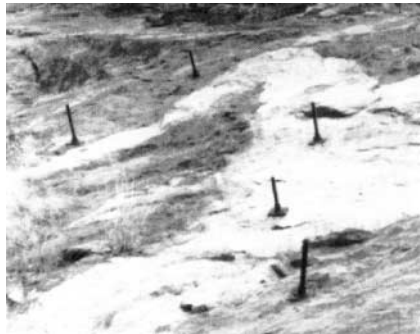
Rock bolts on a rock face
