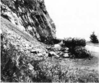
Catch ditch with gabion catch wall
