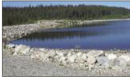
An unprotected reservoir and canal providing drinking water to a community.
