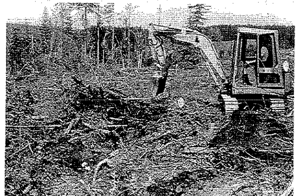
Figure 3. Takeuchi TBO35 excavator.
