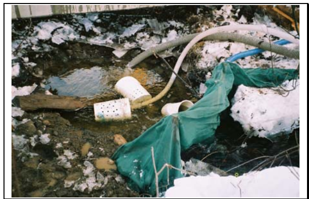
Photo 3. 3000 Road-Site 13/1722, Sumphole at u/s end of in-stream work site.
