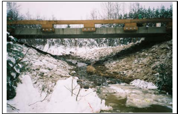
Photo 2. 3000 Road-Site 13/1722, u/s view of reconstructed stream channel (Nov.9/06).
