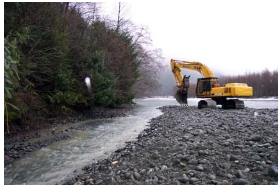
Photo 3 Upstream view of completed channel
