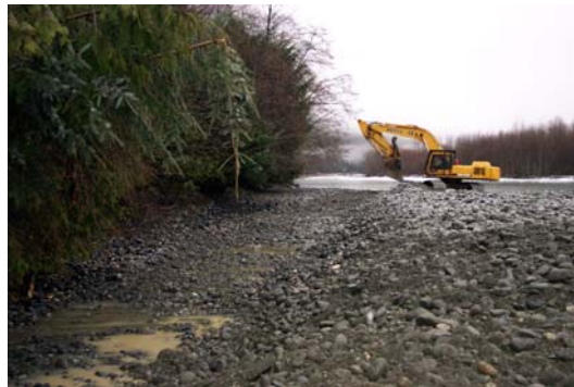
Photo 2 Construction of connection channel
