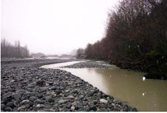
Photo 4 Downstream view of completed channel
