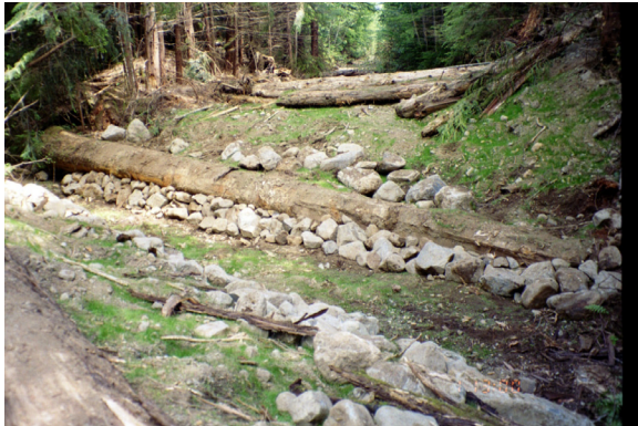
Photo 1. Re-Established, S4, ephemeral stream, utilizing large Cw crib log and rock for armouring.
