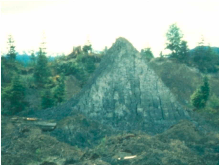
Figure 4. Remarkable, horizontally banded prism slid along a nearly level, to slightly dipping, failure plane. Prism is approx. 4.5 m high.
