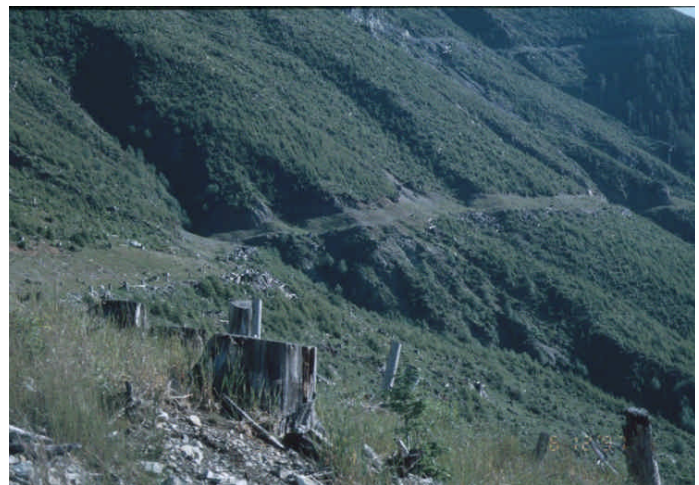
Figure 8. Full deactivation (recontouring) of a forest road.
