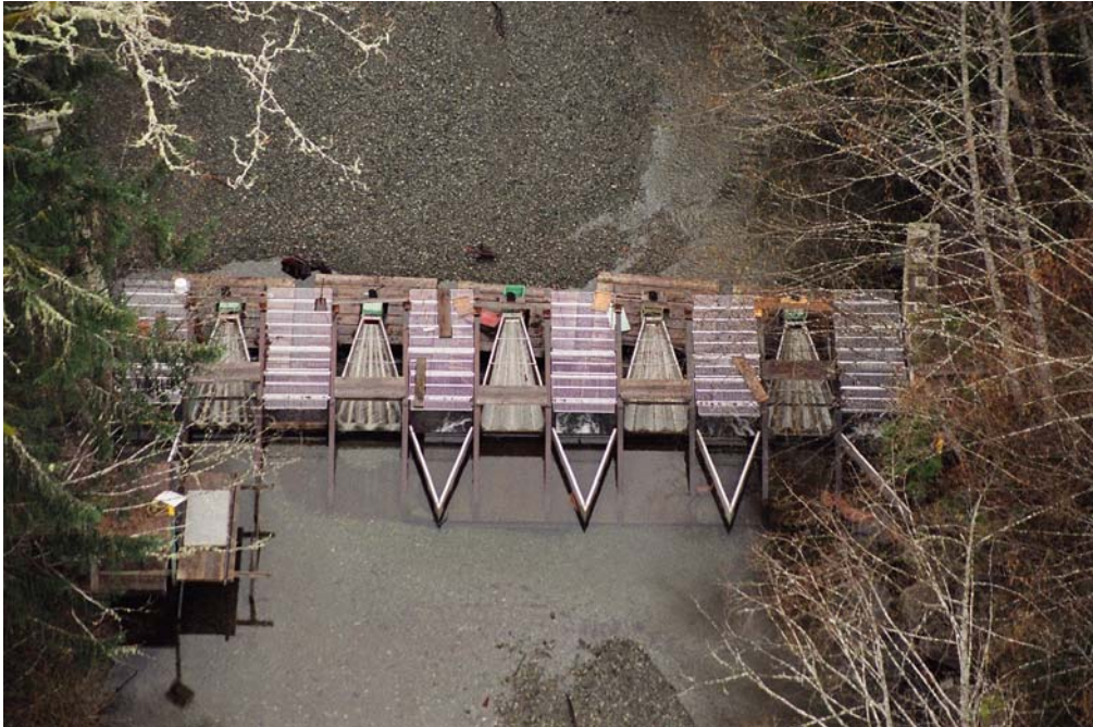
Aerial view of main fish fence located at the head of tidal influence, March 2004. The fence is configured with fan traps for intercepting all juvenile salmon migrating seaward in spring.
