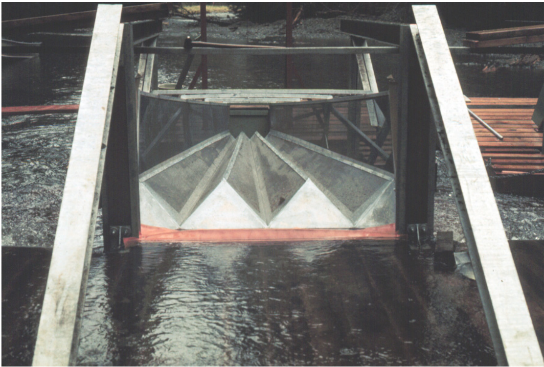
Perforated fan traps direct seaward migrating juvenile salmon into trap boxes at the fish fence.
