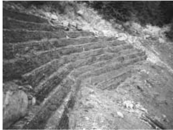
FIGURE 62 Repaired Summit Lake FSR (D. Nicol photo).
