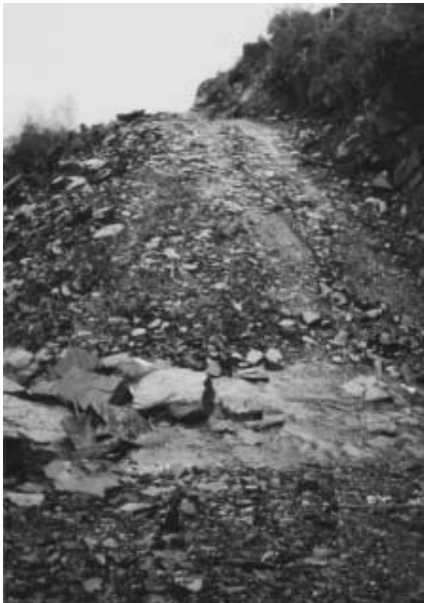
FIGURE 21 Armoured cross-drain on a semi-permanently deactivated road in the Three Arm Creek sub-basin (A. Hasanen photo).
