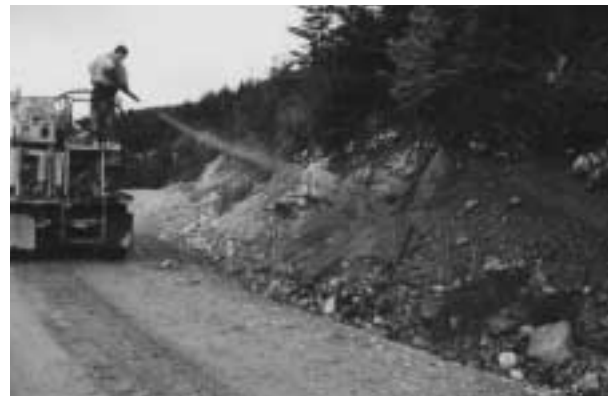
FIGURE 22 Hydroseeding exposed road cutslopes in the Lens Creek sub-basin (A. Hasanen photo).
