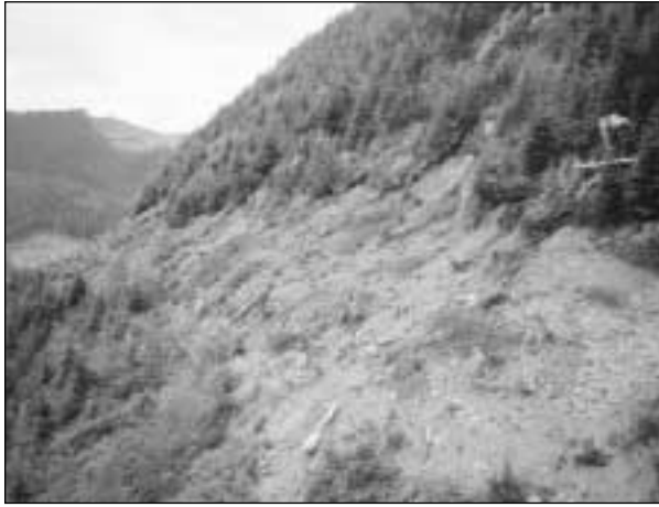
FIGURE 3 Example of road deactivation to reduce probability (likelihood) of landslide occurrence (M. Wise photo).
