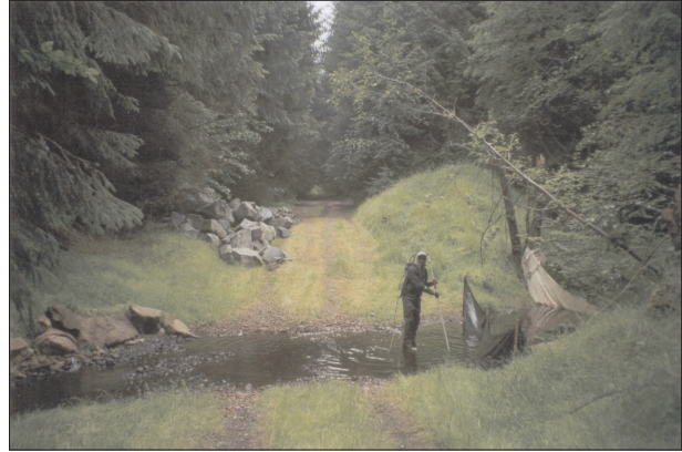
Fig. 8.01 Fish salvage is necessary when conducting work in and about fish streams.
