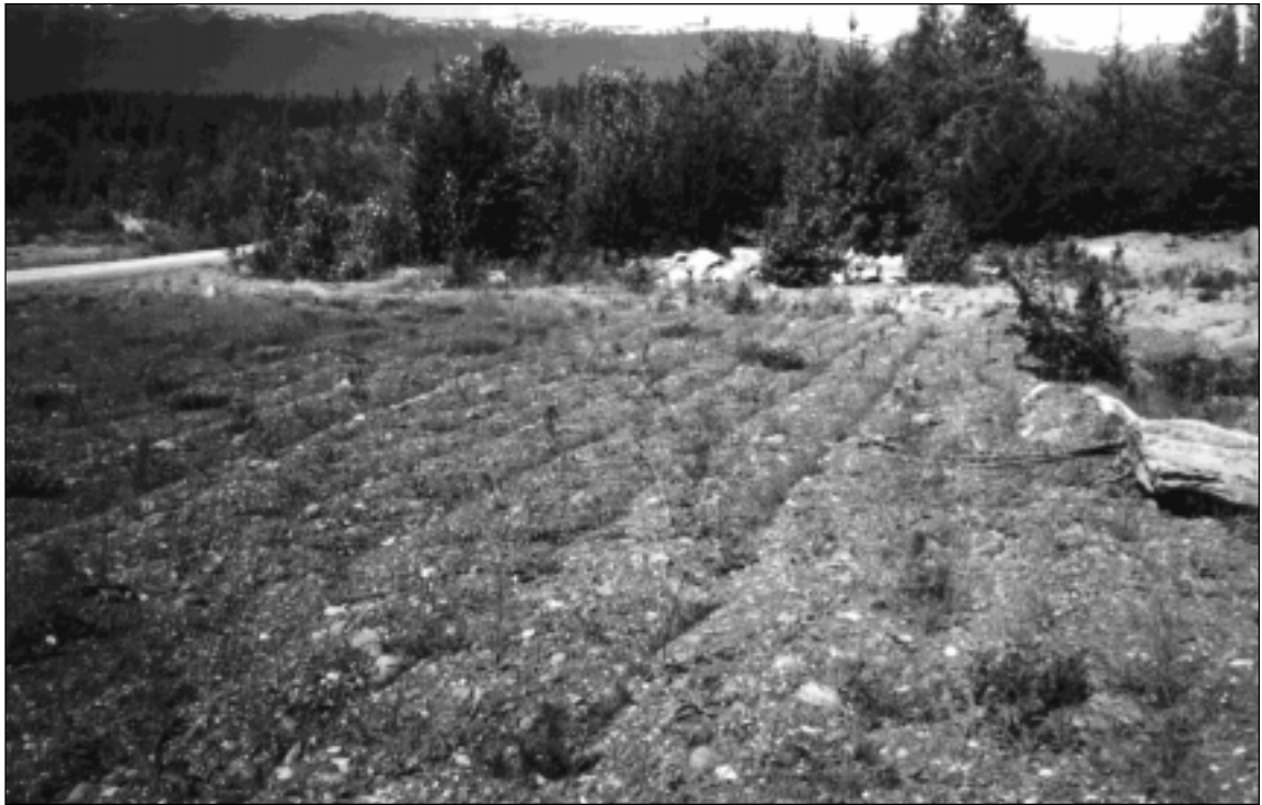
FIGURE 11 Topsoil piles commonly found adjacent to bladed areas on level ground (Kalum Forest District). Respreading these piles should enhance site nutrient conditions and improve productivity.
