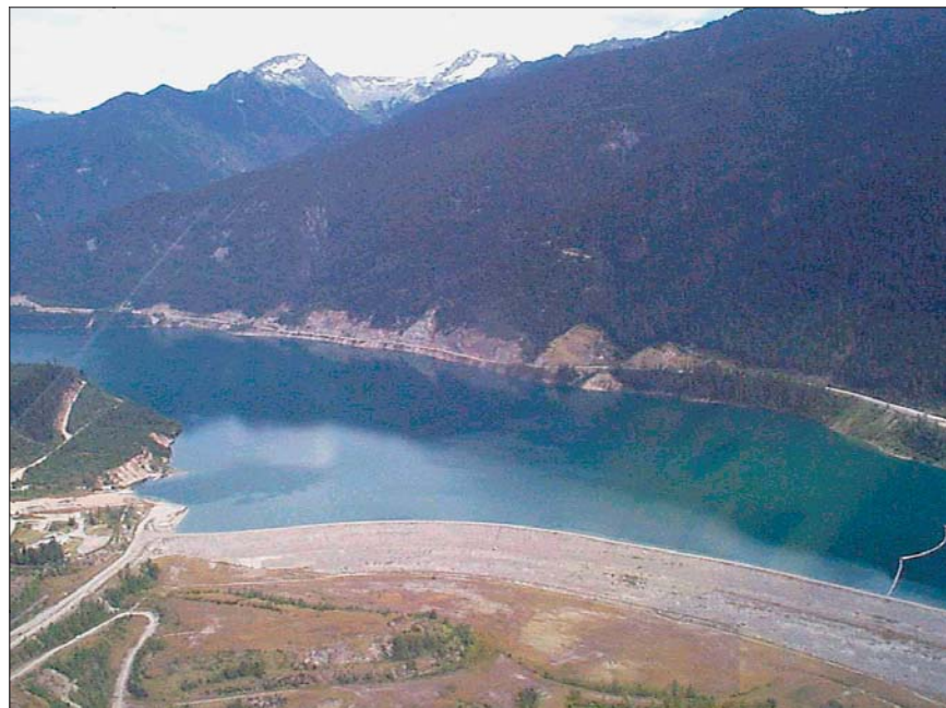
FIGURE 2 Oblique view of slope. Checkerboard Creek enters reservoir at right of main rock cut in centre of photo. Main slope area is to left of creek. Note Revelstoke Dam (earthfill section) in foreground.
