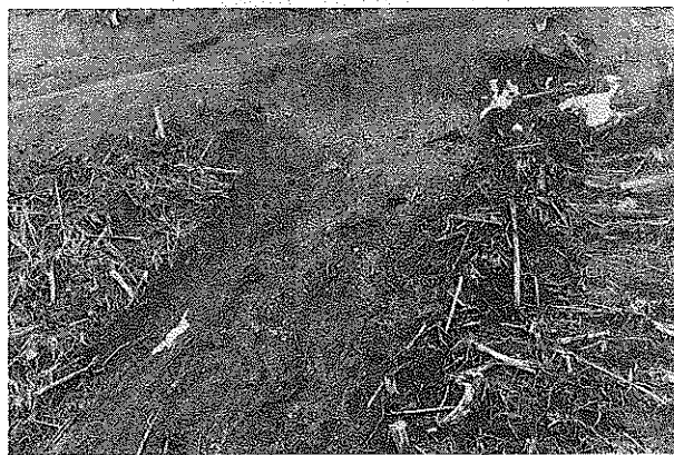
Figure 5. Debris avalanches occur on roads as a result of excess sidecast piling waste material on the outside of a road edge, and inadequate road drainage.
