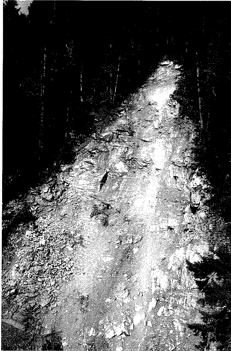
Photo 3 (DFV98/02/09/1-21) Front view of Slide A showing the material exposed on the failure plane.
