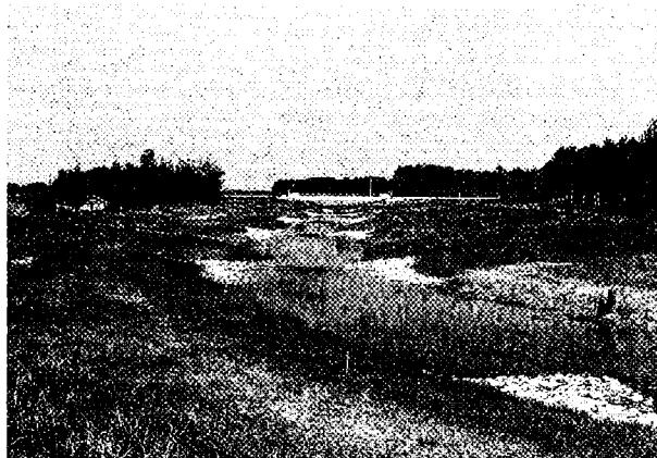
Fig. 9 Fieldstone riffles added to the lower Mink Creek channel. The riffles continue to impound shallow pools under low-flow conditions after the spawning season, facilitating the return of drifting fry to the lake downstream.
