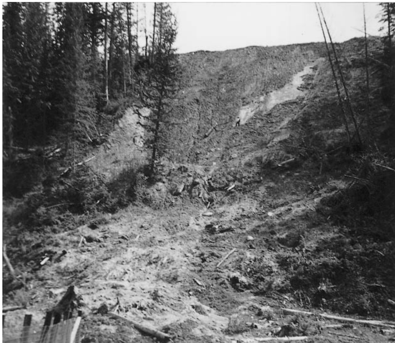
Fig. 6. Morkill 31.5 km (see Fig. 2 for location). Earth slide in sandy soil below an abandoned cutting permit access road.
