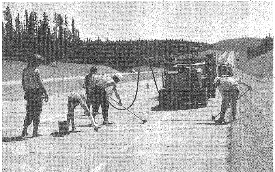
Road crews apply Infratech Polymers Inc.'s road crack sealant — a Canadian market of 18 million linear metres annually
