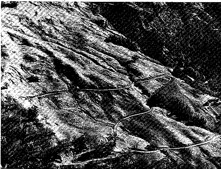
Figure 4-c. Massive slope failure in the northern California Coast Ranges. The failure has resulted from creep and progressive failure in a deeply weathered series of greywackes, shales, bedded cherts, and limestone lenses of Cretaceous Age.
