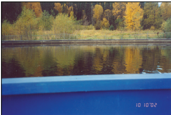
Plate 2. A settling pond located beside the Upper Fraser pump house.
