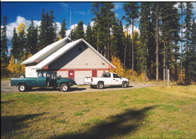
Plate 1. A view of the Tumbler Ridge water treatment plant. The raw water samples were collected from an inside tap.
