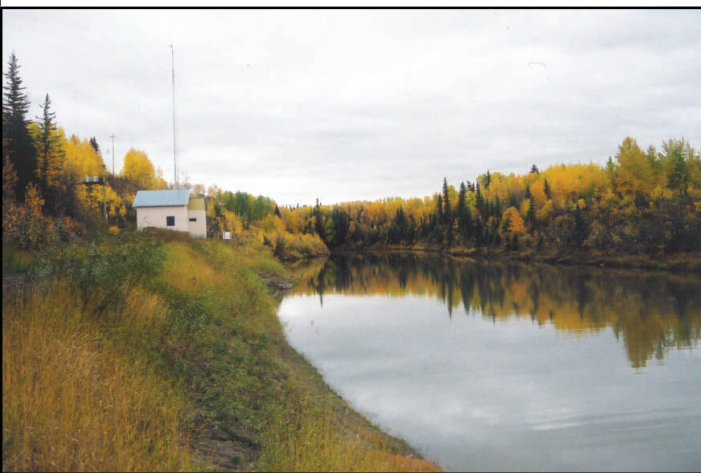
Plate 1. An upstream view of the Kiskatinaw River (from the cross-channel weir) and the Dawson Creek pump house.
