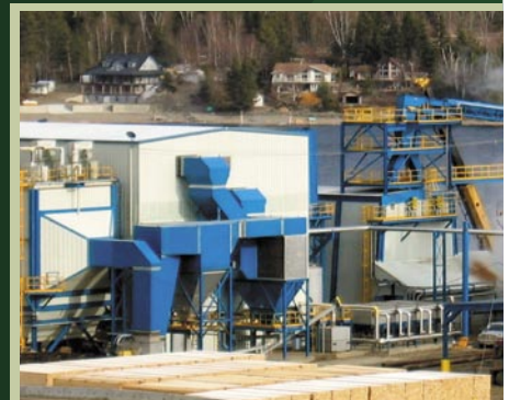
New thermal energy system at Interfor's Adams Lake sawmill.
