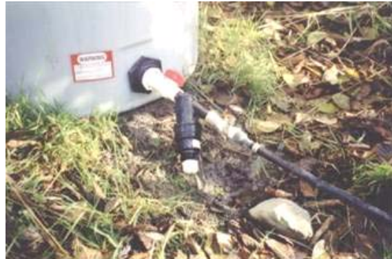
Figure 1. Drip-tank with valve and filter.
