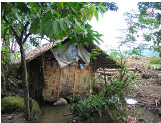
Figure 4. A house remains mostly intact near the edge of the landslide.
