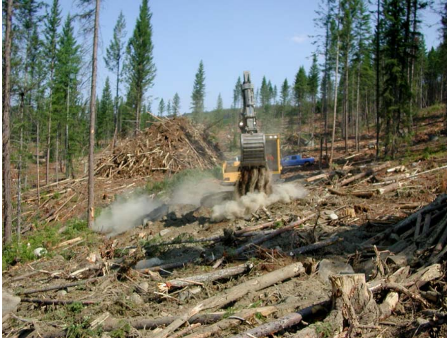
Rehabilitation of a temporary road
